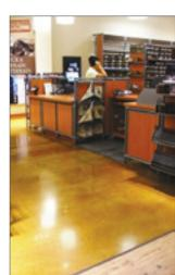
All Lythic™ products increase the strength and durability of concrete with each application. Utilizing colloidal silica, Lythic™ Densifier improves concrete as it bonds quickly and cleanly with calcium hydroxide components in all concrete.
