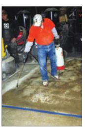
sized particles, suspended in an ultra low surface tension liquid, penetrates deeply into concrete surfaces bonding with the cement components of the slab. Lythic<sup>™</sup> Densifier makes an extremely hard, dense floor surface that has increased wear resistance to foot and fork lift traffic. It is water based and environmentally friendly and is VOC compliant in all states.
